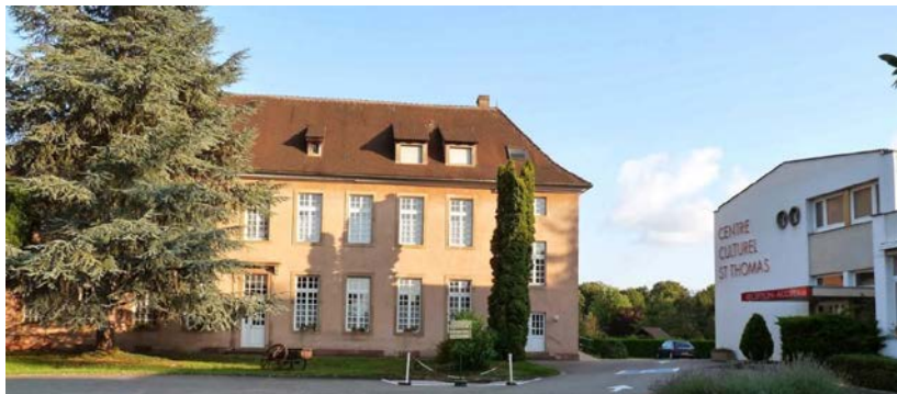
Centre Culturel St. Thomas in Strasbourg (on the right)
